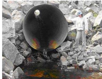
Charlottetown Brook. Depth <1 cm. Drop of 35 cm on to rocks. About 3/4 of the flow was under the culvert. High gradient. We saw four ~12 cm trout in the pool at the outlet. Small streams similar to this one are important rearing areas for small salmon and trout, but such improperly placed culverts obstruct migration.
