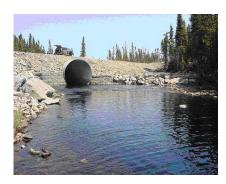
Inlet of the pipe culvert at Shinney's Brook, installed on a previous riffle area. The culvert is not properly sized for the stream, is not embedded and creates a velocity barrier for upstream migration of small fish. Salmon spawning and rearing habitat (442.6 m<sup>2</sup>) and riparian vegetation has been lost. A bridge spanning the river should have been built here.
