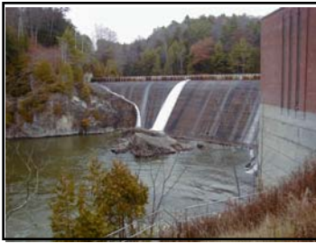
Peterson Dam as seen from down-
